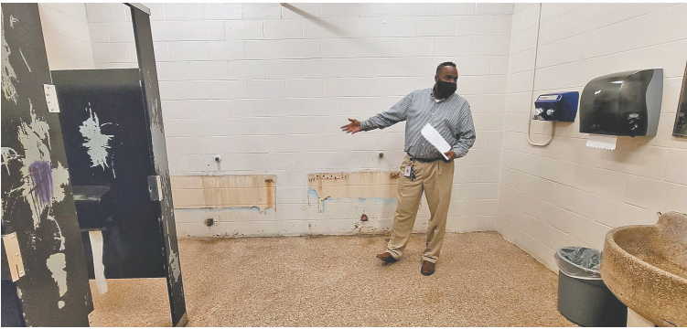
FILE PHOTO BY R. HANS MILLER RISD Operations Director Derrick Dabney shows where urinals are missing from the walls in the boys’ bathroom and Royal Junior High School. Collapsed drainpipes in the walls and under the floor have prevented the installation of new urinals – one of many serious maintenance issues at the half-century-old campus that the district hopes to fix via a bond election this fall.
