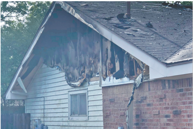
The lightning strike caused a fire and a transformer explosion.
