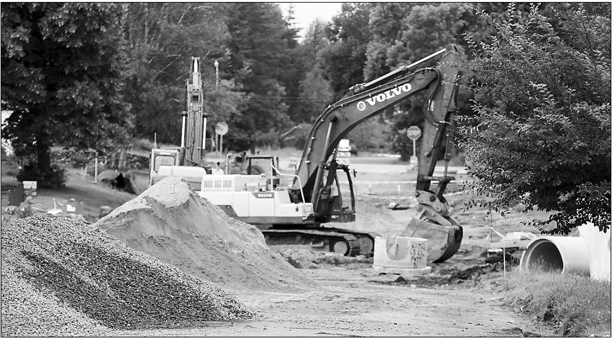
Road construction crews are working this summer on reconstructing a portion of Pattison Street in Ely, between Central and Third Avenue. New water and sewer pipes, and sidewalks, are part of the project. photo by K. Vandervort
