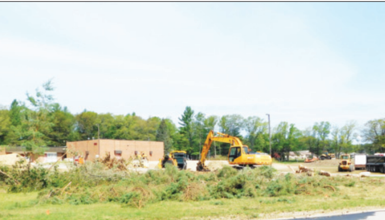
Grade and substrate work is underway on the Larson Elementary School expansion project, starting with removal of the topsoil. (Cleaver photos by Dianne Alward-Biery)
