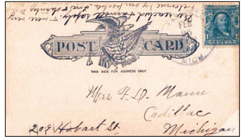
Postcard of the Portland Cement Company (front above, top-back above, bottom.)
