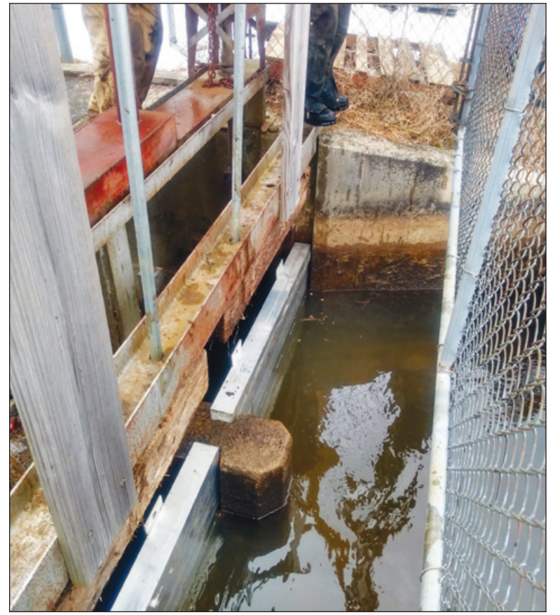
These photos show the replacement work done in early 2020 to replace the 50-year-old stop logs with new aluminum stop logs at Doc and Tom Lake/Lake of the Pines in Freeman Township. (File photos courtesy Carl Parks)
