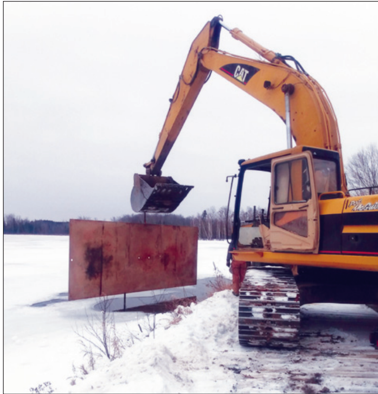
These photos show the replacement work done in early 2020 to replace the 50-year-old stop logs with new aluminum stop logs at Doc and Tom Lake/Lake of the Pines in Freeman Township. (File photos courtesy Carl Parks)
