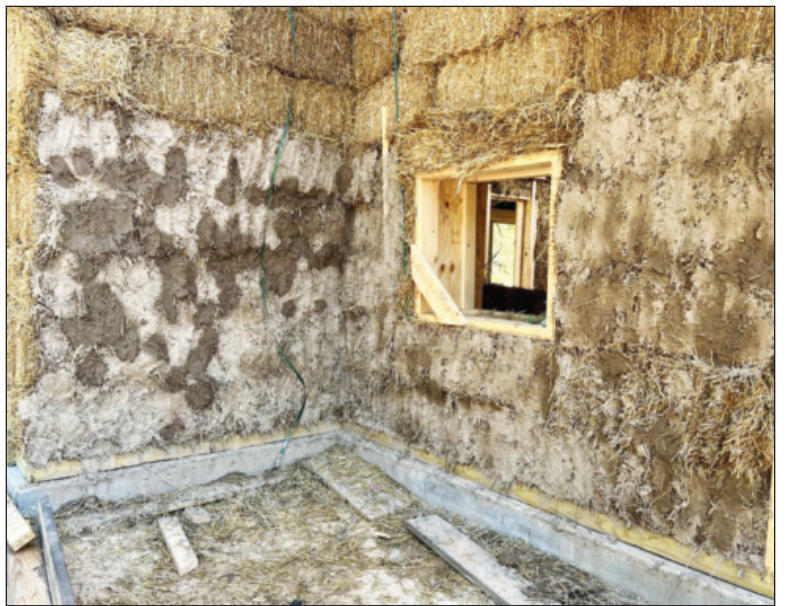
View of the interior ground floor of the straw bale home. The home will be an open concept home to allow for familial cohesiveness and interaction. The photo below shows the work Mara Kalat-Brown had just started by applying the initial layer of clay-based plaster to the straw bales. That plaster consists of clay sand and fine straw. (Cleaver photos by Megan Barron)
