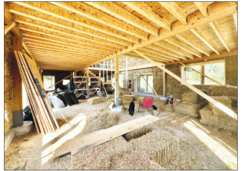
View of the interior ground floor of the straw bale home. The home will be an open concept home to allow for familial cohesiveness and interaction. The photo below shows the work Mara Kalat-Brown had just started by applying the initial layer of clay-based plaster to the straw bales. That plaster consists of clay sand and fine straw. (Cleaver photos by Megan Barron)
