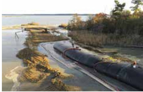
The Barren Island restoration process could be seen underway in October 2025 in drone photos (SUBMITTED PHOTO)
