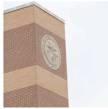
SCOTT W. COLEMAN The Leander Independent School District Administration Building at 204 W. South Street in Leander, Texas.
