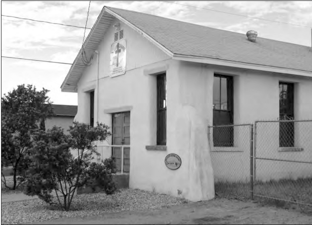
Phillips Chapel Christian Methodist Episcopal Church after volunteers, including faculty and students from NMSU and Dona Ana Community College, spent seven years restoring the historic church. (Photo by Beth O'Leary)
