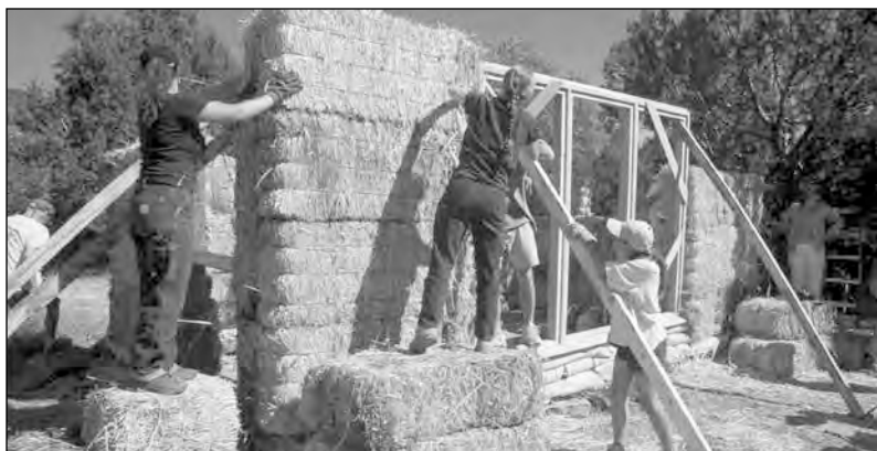
Volunteers with Builders Without Borders raise a straw bale wall. (Courtesy Photo)
