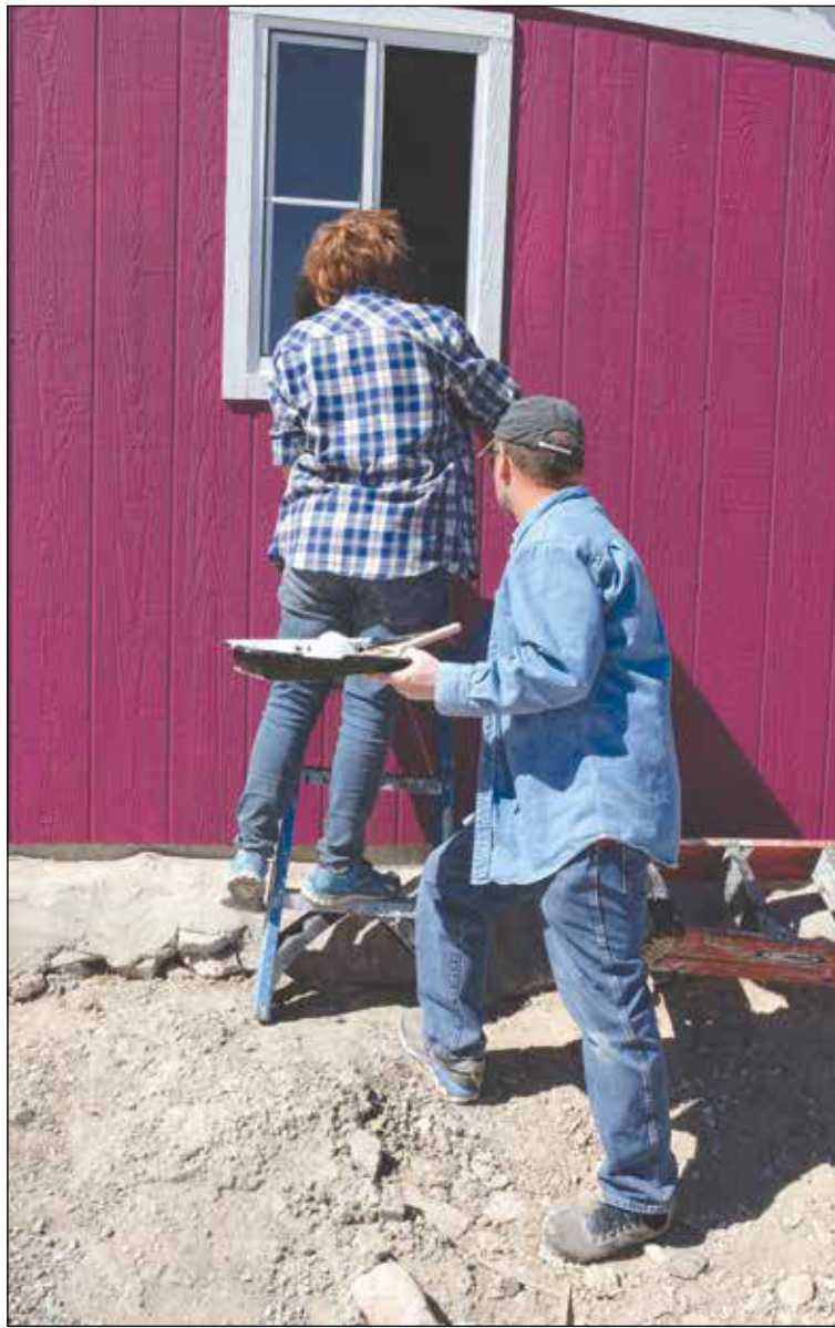
Pete, on the ground, and Terry Frank from Las Cruces work on the house in Juárez.
