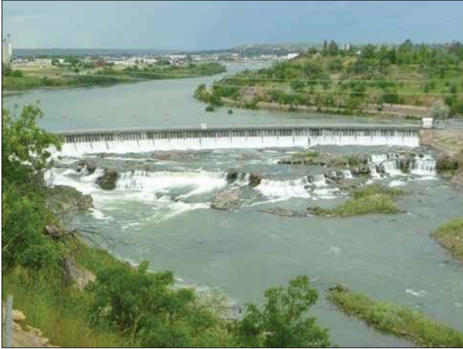
One of the water falls along the Missouri that Lewis and Clark once had to skirt which is still going strong. "We loved Great Falls Montana for its friendly folks, history and small town atmosphere," Sonne said. (Photo by Lee Sonne)
