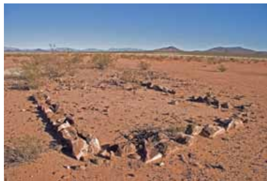
Primitive foundation for early house on the arid Jornada del Muerto, where settlers struggled daily with the needs for water.
