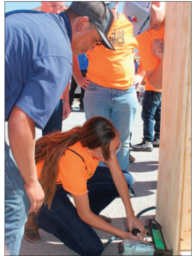
Ciara Quezada hammers in a sidewall in the Oñate High School shed, with support of Carlos Valenzuela of Veloz Homes.
