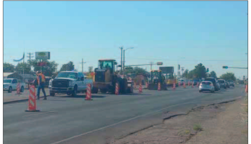
Construction on the $23 million Valley Drive renovation project began June 25.
