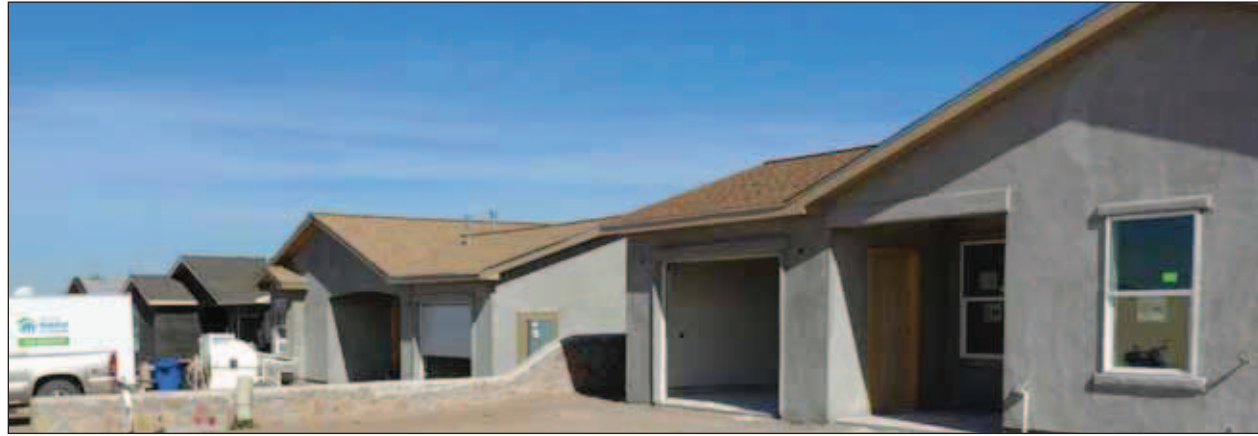
H4H houses under construction on Aurora Star Court.
