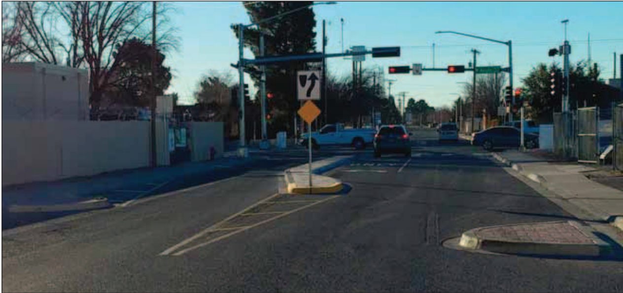
Traffic calming on Melendres Street near Amador Avenue includes the curb extension, called a choker, and a raised median.
