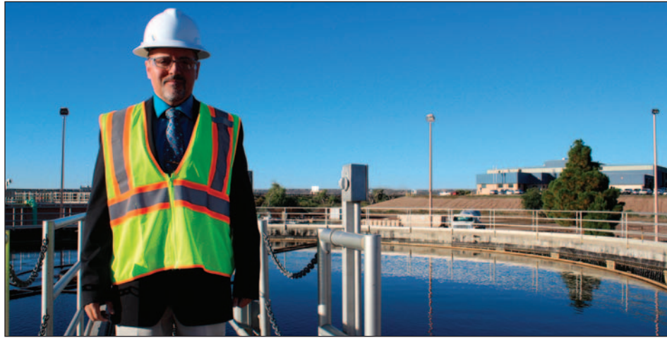
John Mrozek, the new LCU Wastewater administrator, pauses on the walkway across the top of one of the primary clarifiers at the JHWWTf.
