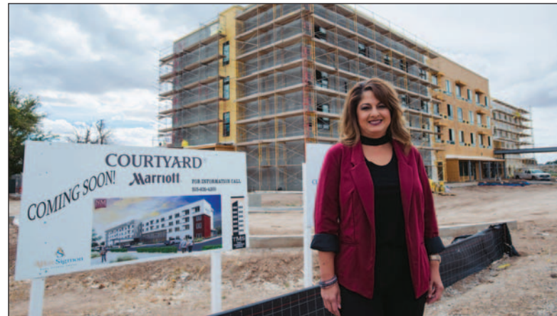
Amy Miller stands in front of the partially completed hotel.
