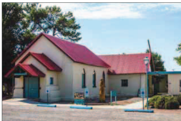
St. James Episcopal Church parish hall in November 2017, with almost all renovations complete.
