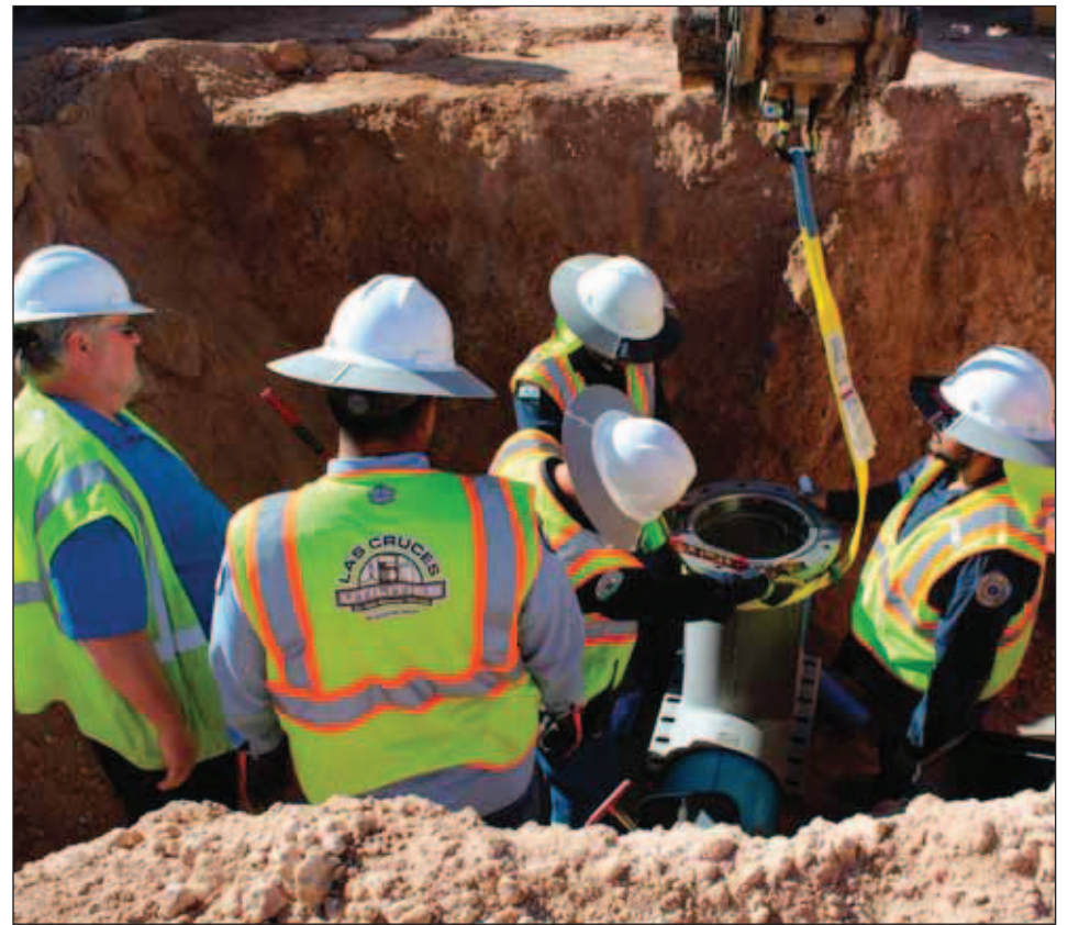
An LCU crew mounts the housing for the drill that will be fitted onto a "live" underground water pipe.
