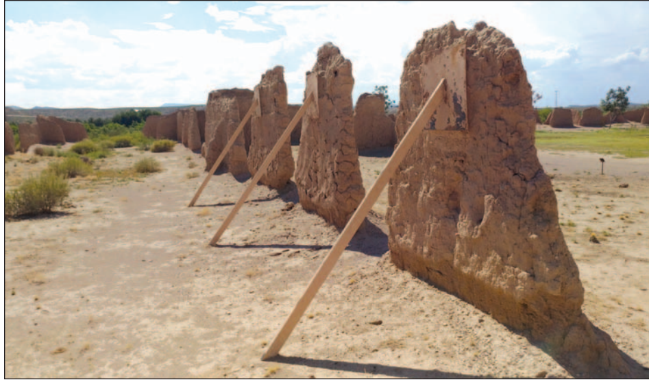
Efforts continue to preserve the adobe walls of Fort Selden historic structures. The adobe bricks used to construct the fort have a high sand content, making them vulnerable to wind and rain erosion.
