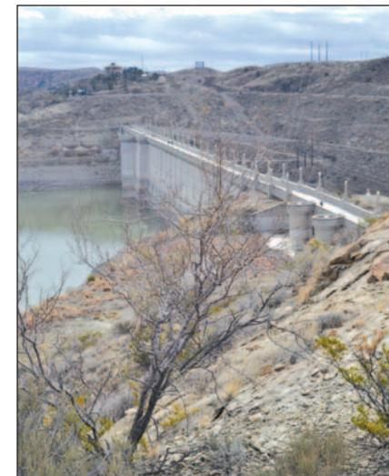
Elephant Butte Dam turned 100 years old in 2016. At the time the dam was built, it was the largest concrete structure of its type in the world. The structure is 301 feet high and the road on top is 1,162 feet long.
