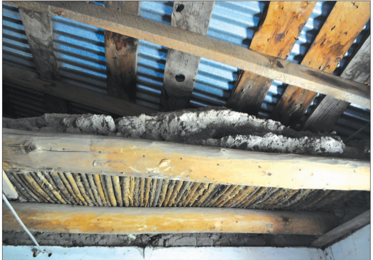
ABOVE: Latillas of sotol set across beams and topped with mud were found above the ceiling in one of the rooms of the Black Range Museum, formerly the Ocean Grove Hotel.
