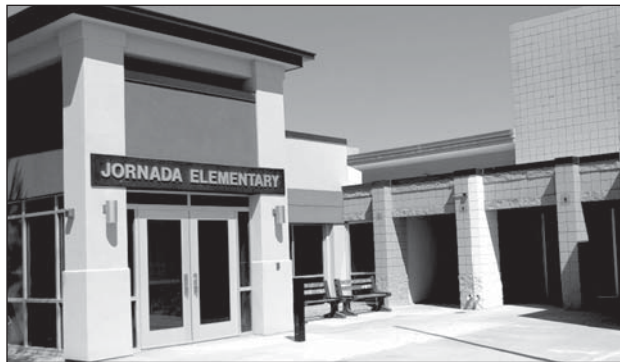
The front office and main entrance are being relocated at Jornada Elementary School.
