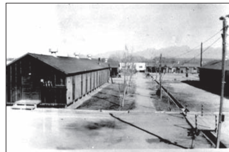
The barracks of the HSR office, 535 S. Melendres St., when it was a Civilian Conservation Corps (CCC) camp.
