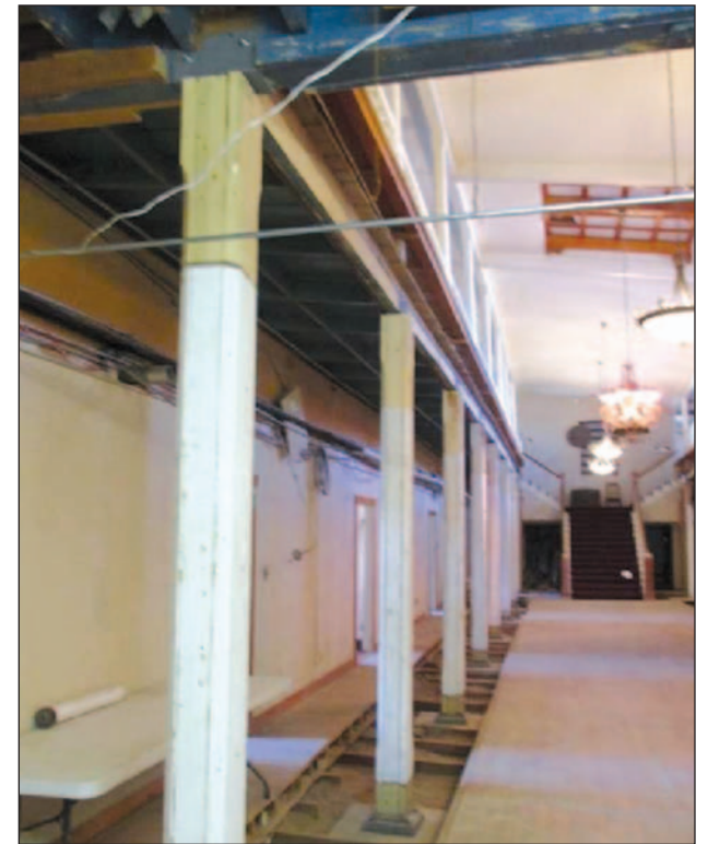
Columns completed on the east side of the hotel lobby.
