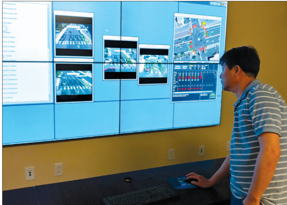
City Traffic Operations Engineer Soogyu Lee monitors (and can adjust) traffic flow on the media wall at the city's Traffic Management Center on Hadley Avenue.
