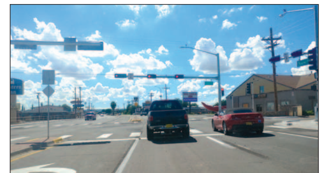
The city has installed a new traffic signal at the intersection of Picacho Avenue and 17th Street.
