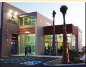
Southwest Center on Aging gets new office B29
