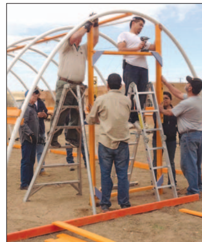
Participants in the Southern Pueblo Beginning Farmer and Rancher Program assemble a hoop house during a workshop provided by New Mexico State University's Rural Agricultural Improvement and Public Affairs Project.
