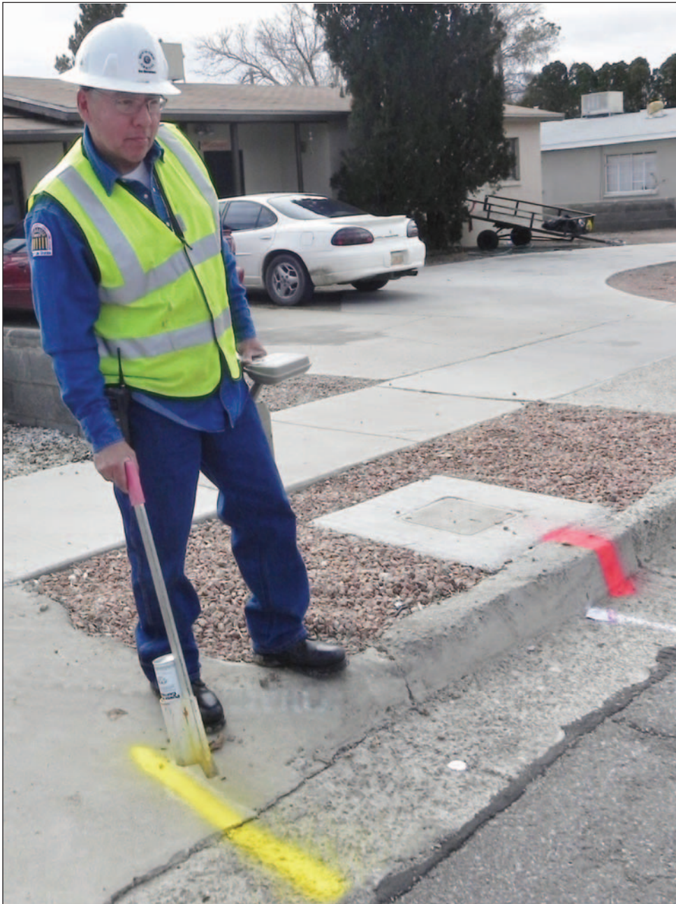
LEFT: When you dial 811, a locator will respond and mark all underground utilities by specific color – up to the meter on your property – to indicate where the pipes are located. Generally the gas meter is located right next to the home or office.
