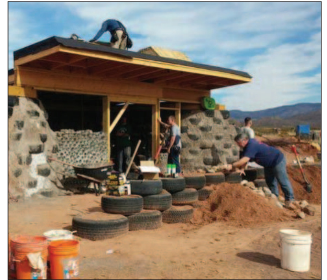
A foxhole house being constructed out of recycled and repurposed materials.
