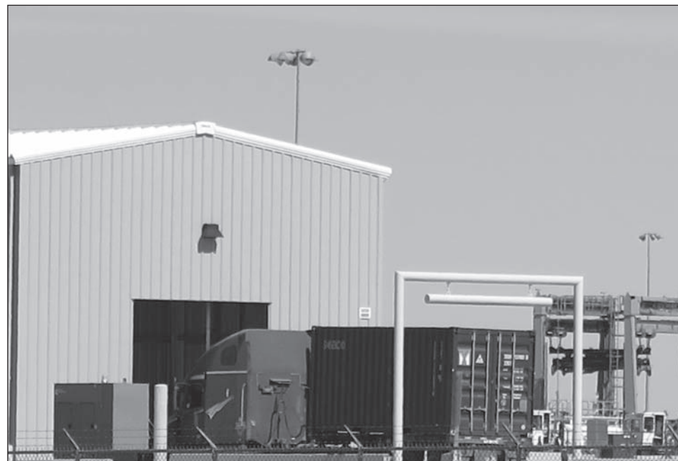
The Union Pacific intermodal facility.
