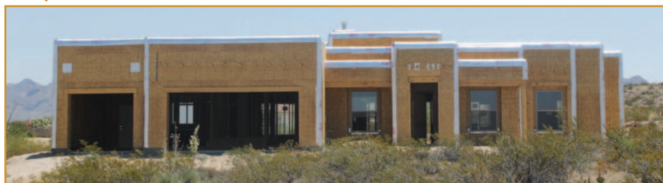
The house in its “roughed-up” phase.
