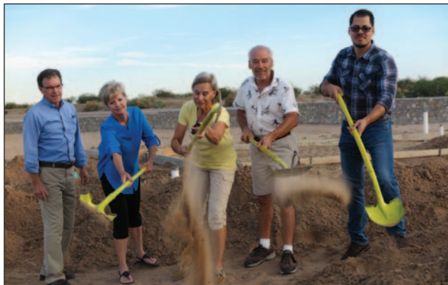
With Bob Pofahl watching, Karen Pofahl, Ann Clark, Tom Clark and builder Javier Cabrera of NetSolar Homes hoist some dirt at the groundbreaking for The Willows at Picacho Mountain courtyard home community Oct. 28.
