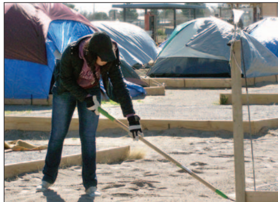
New Mexico State University student Melissa Gonzales spreads loose gravel on the walkway between plots at Camp Hope to help prevent puddles and mud bogs from forming. NMSU students from Engineering Without Borders volunteered at the camp during the spring 2015 semester.
