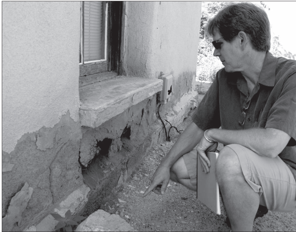
Mesilla Valley Preservation, Inc., President Eric Liefeld indicates coving typical of subflorescence, where expanding salt crystals destroy adobe pores on a microscopic level.
