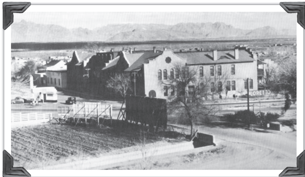
New Mexico State University Library Rio Grande Historical Collections photo Loretto Academy, built in 1907 by Trost & Trost, sat at the south end of Downtown Main Street until it was demolished in 1959.
