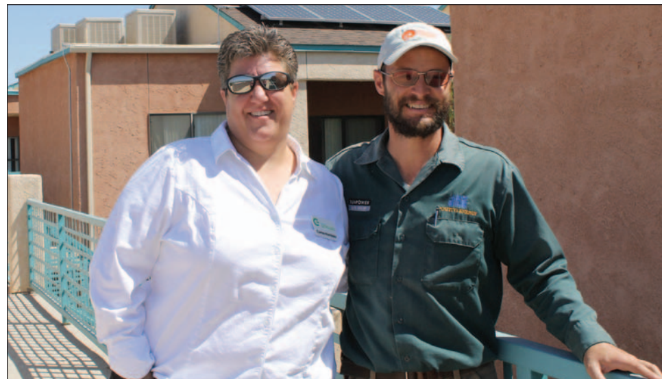
Las Cruces Green Chamber of Commerce Executive Director Carrie Hamblen and Las Cruces branch founder of Positive Energy Solar Mark Westbrook survey the 29-kilowatt solar array installed at Regency Pointe Apartments, 3000 Maestic Ridge, during the system's ribbon cutting ceremony Wednesday, June 4.
