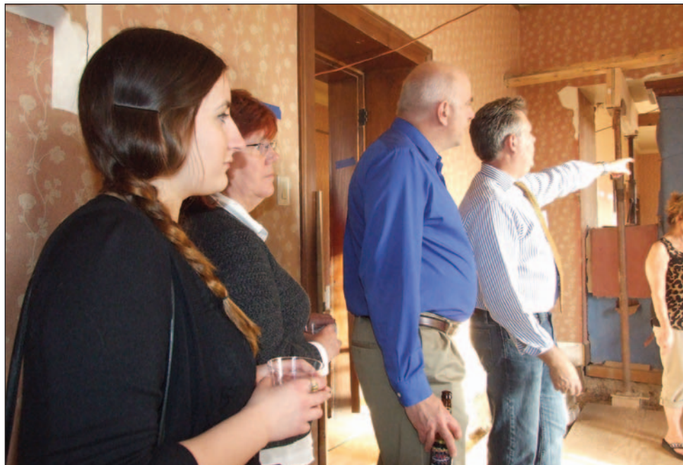
Bill Allen, president and CEO of the Greater Las Cruces Chamber of Commerce, points out to attendees at the Thursday, March 27, Business After Hours work being done on a new HVAC system for the Nestor Armijo House, 150 E. Lohman Ave. The chamber is restoring the 19th century structure as part of a complex that later will include a new chamber office building.
