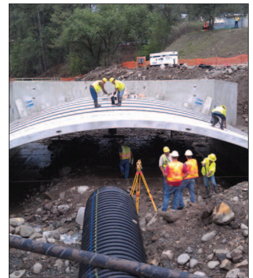
Zia Engineering conducts a construction inspection for the Eagle Bridge project.
