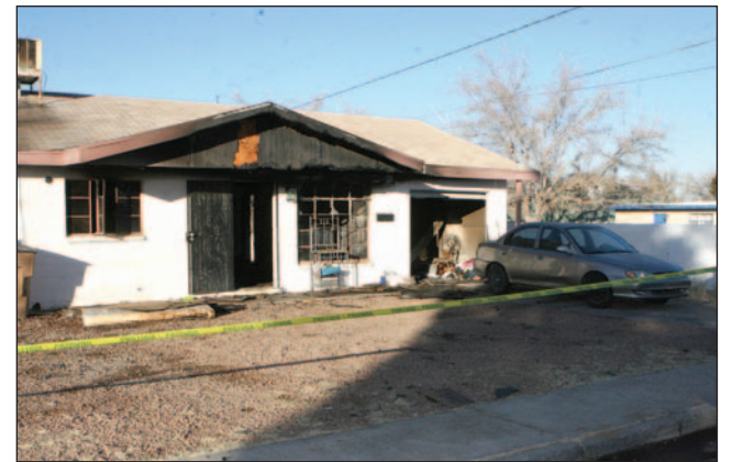
The burned home, which stands at 1304 Thomas Drive
