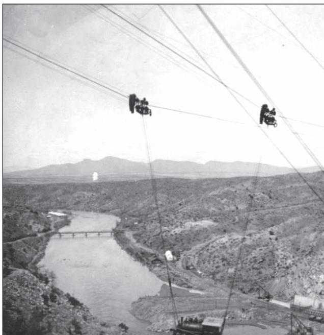
A grab bucket dumps sand into railroad cars Oct. 29, 1912.
