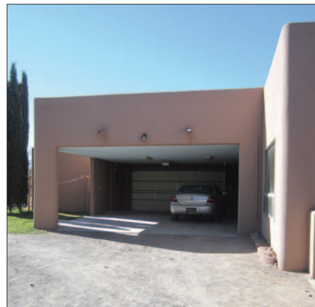
The back side of the garage is open on two sides, allowing the area to be used as a covered patio.
