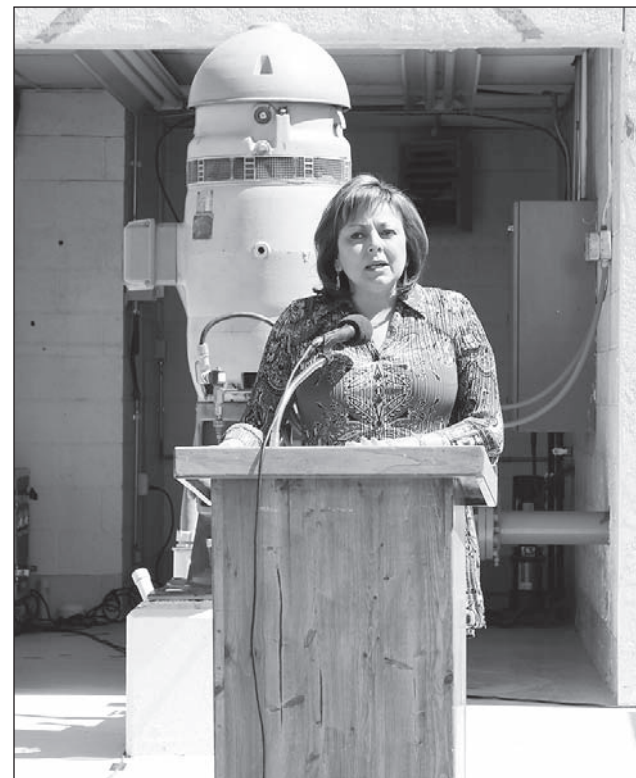
Martinez announces the City of Las Cruces getting $4.25 million for water infrastructure in front of 37-year-old pump No. 32 near Munson Senior Center Tuesday, April 8.
