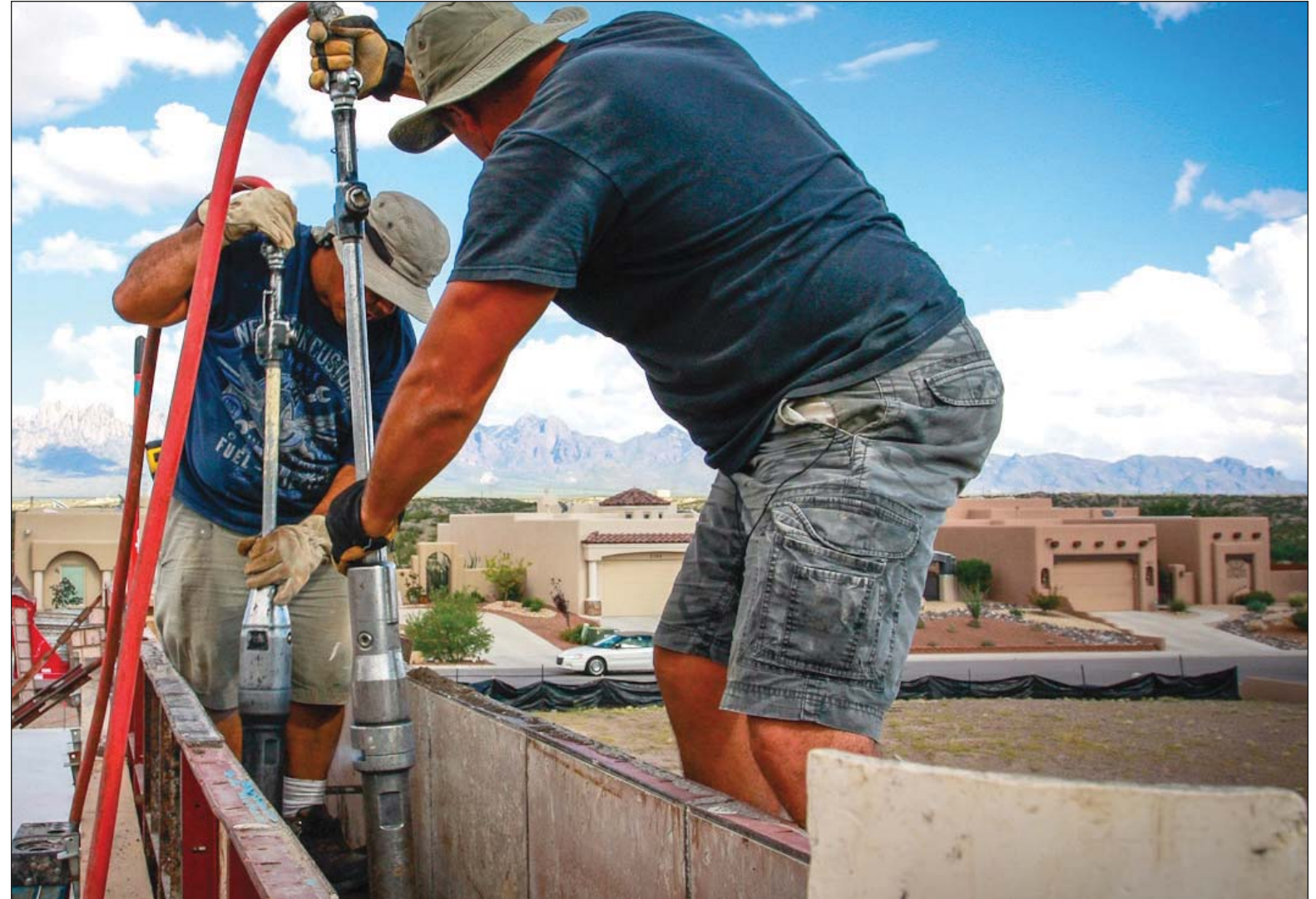
Raul Muro, left, and Chuy Casteneda use a pneumatic tamper to work on a wall for a rammed earth home for Soledad Canyon Earth Builders.
