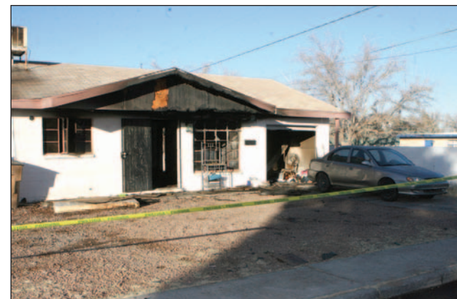
The burned home, which stands at 1304 Thomas Drive
