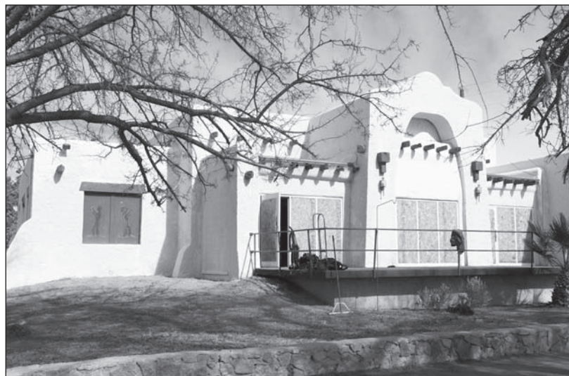
The Las Cruces Country Club clubhouse, recently confirmed to be of Trost design, will be one of several historic buildings featured in the Casas de Antaño tour from 1 to 5 p.m. Saturday, Feb. 15.
