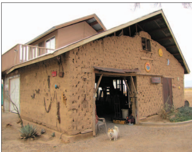
An original adobe façade wraps around the modern pole barn, which has an upstairs studio and balcony.
