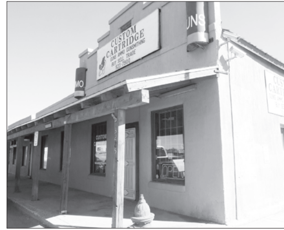
Commercial buildings on Main Street in Mesilla Park run the gamut from highly functional to in need of serious rehabilitation.
