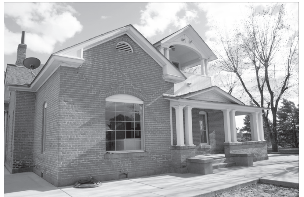
The C.T. Turney House, located on Boutz Road, was built by one of the biggest ranchers in Doña Ana County. It is one of eight homes featured during the tour that demonstrate adaptive reuse.
