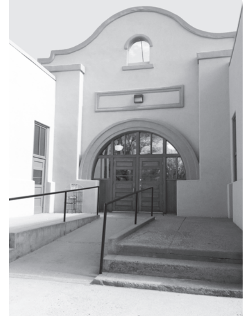
The Mesilla Community Center – once the Mesilla school – will be a stop on the historic home tour.
