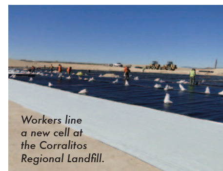
A worker uses heavy equipment to compact trash at the landfill.
