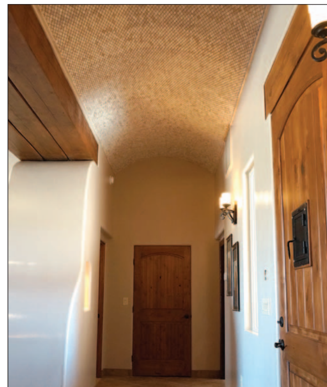
Tile covers a barrel arched hallway ceiling.
