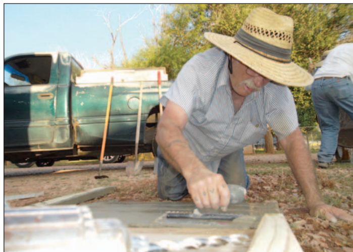
Dave Coshnet smooths out the cement foot of the ramp.
