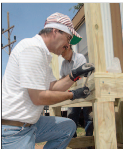
Mark La Fountain tightens lag bolts on the larger porch.
