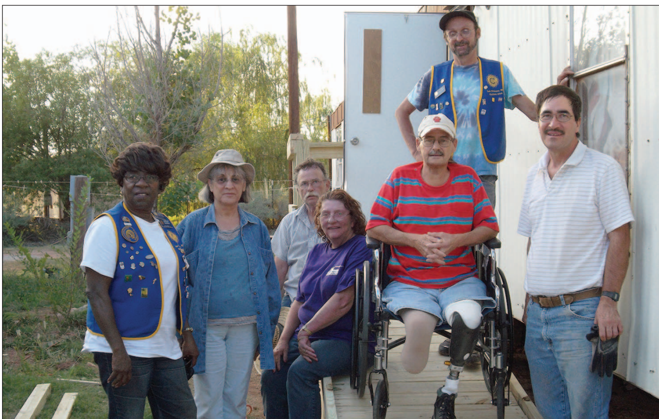
Las Cruces Civitan members pose with Langley on the nearly finished ramp.
