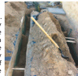
400' Copper Tubing Install
